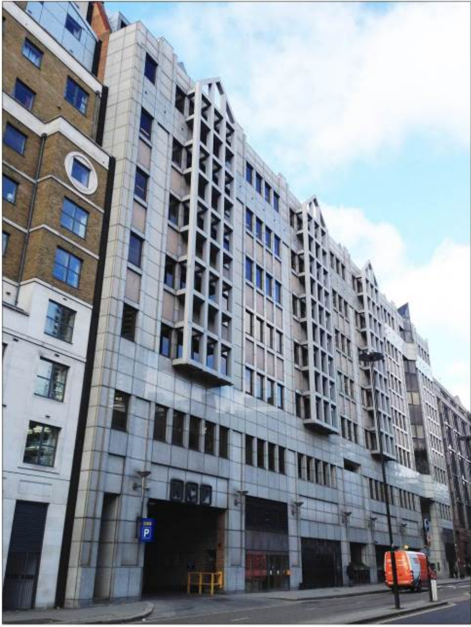
160 Aldersgate Street, view from south east
