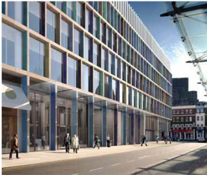
View looking south along Lindsey Street showing proposed building Case No. 13/00605/FULEIA: Farringdon East Crossrail Oversight
